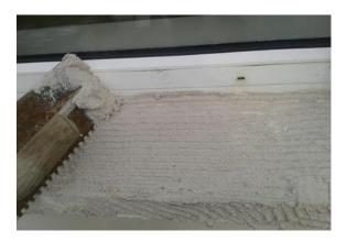
**Step 4:** Using a serrated trowel apply an even coat of adhesive over the old sill. Also place adhesive on inside front face of new sill and put into place.
