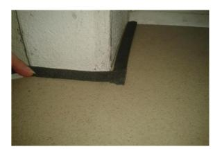
**Step 5:** Apply Passive Sills sealing tape at either side of the sill to take reveal boards. (If the reveal is stepped the Passive Sills sealing tape needs to overlap on the corner.)
