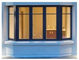
**Step 8:** If desired, acrylic finish or masonry paint can be applied to finished sill.
