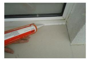
**Step 6:** Run a fine line of polymer sealant between the window and the sill.
