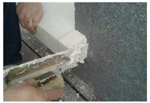
**Step 7:** Apply Passive Sills repair mortar to cut ends.
