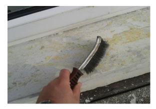
**Step 1:** Remove any dirt, debris, loose paint, algae etc. from the old sill with a wire brush.
