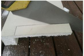
**Step 2:** Cut new sill to size using a fine tooth hand saw allowing a 5mm gap at the back of the sill to allow for Passive Sills sealing tape.
