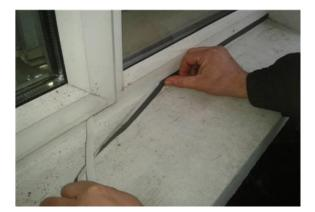
**Step 3:** Apply Passive Sills sealing tape to bottom of the window frame.
